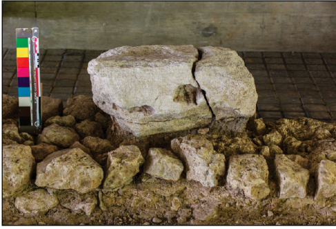
Figure 2. Kunrader limestone blocks forming the foundation of the porticus of the Roman baths of Coriovallum. The rough-hewn blocks are from a local quarry. A Norroy limestone pillar base rests atop them (photograph courtesy of Het Romeins Museum).
